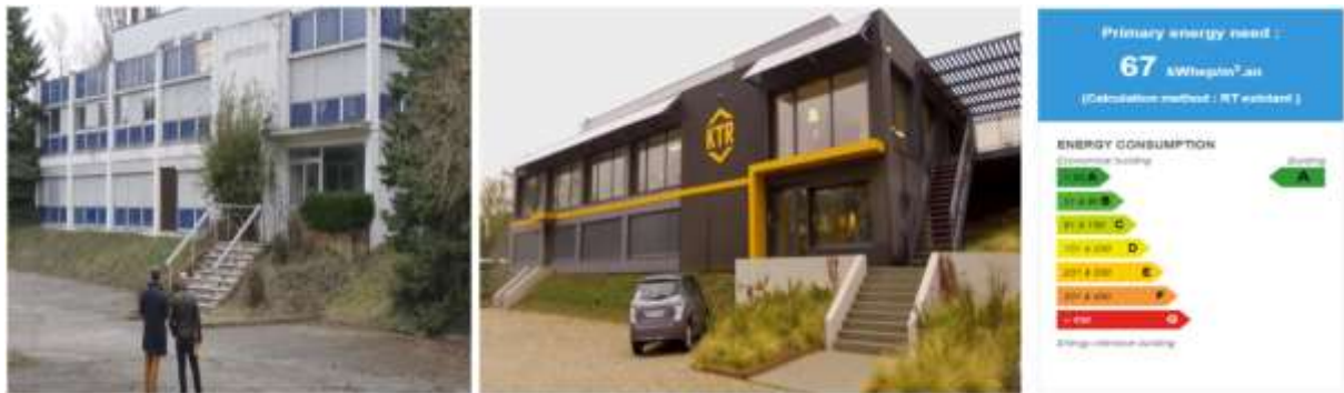
Picture 6. Building Images Before and After Retrofitting (URL-11)
