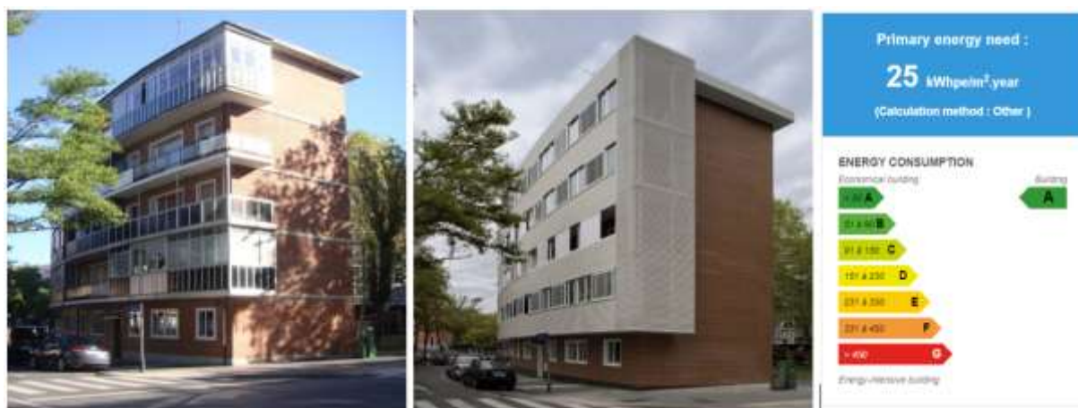
Picture 1. Building Images Before and After Retrofitting (URL-5)
