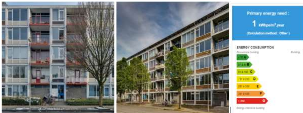
Picture 4. Building Images Before and After Retrofitting (URL-8)
