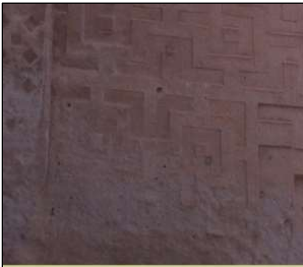
Figure 11. The shapes on the surface was erased with the effect of wind and rain on Midas monument
