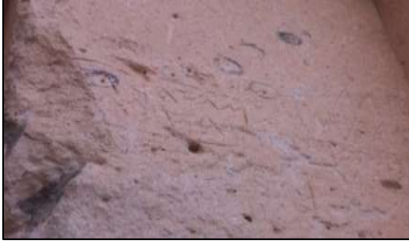
Figure 6. Substance loss on the surface of the Midas monument with a cutting tool
