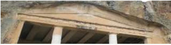
Figure 15. Black stratification observed on the upper surface of the Gerdek rock tomb monument due to atmospheric pollution
