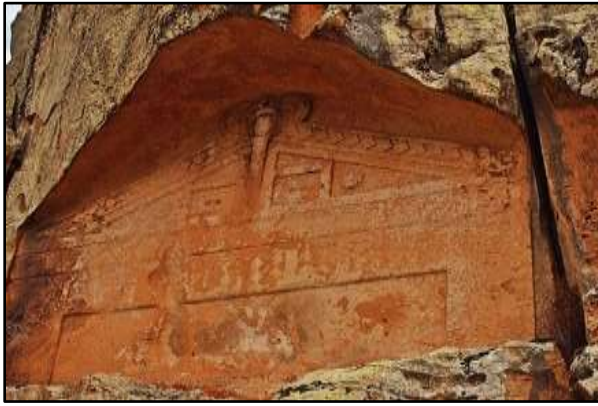
Figure 19. Loss of texture with salt formation on the Bitmemiş monument (Url3, 2019)
