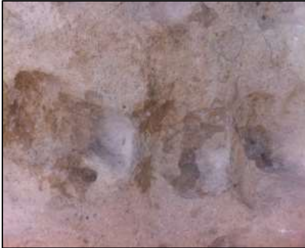
Figure 5. Contamination caused by the accumulation of matter in the cavities formed with the cutting tool on the stone surface
