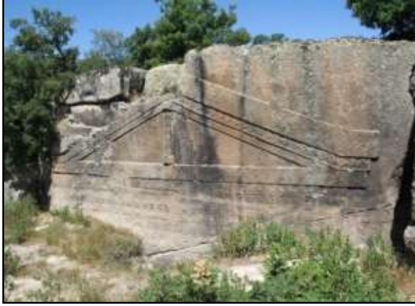
Figure 14. Contamination and black layer formation on the surface of Maltaş monument (Url2, 2019)
