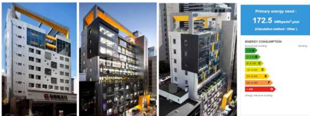
Picture 7. Building Images Before and After Retrofitting (URL-13)
