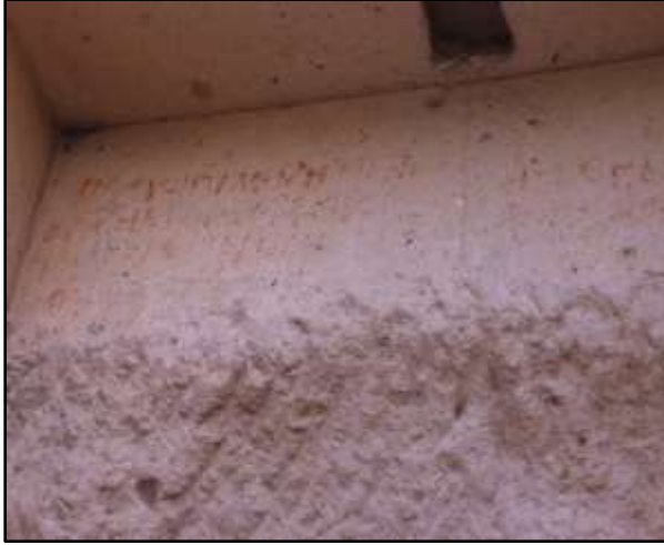
Figure 4. Loss of substance resulting from the operation with a cutting tool on the Midas monument
