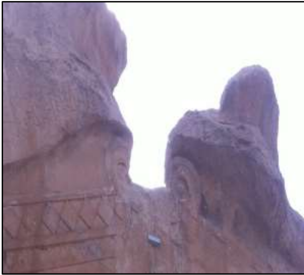
Figure 9. Material loss due to undetectable effect observed in the upper part of the Midas monument
