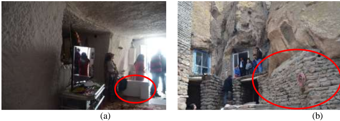
Figure 6. Stone walls used as dividing walls (a) and to support the building (b) in Kandovan (2018)
