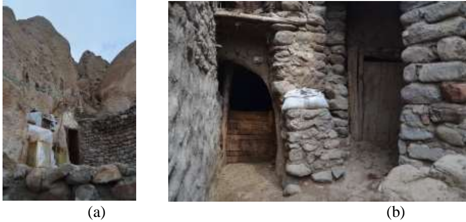
Figure 3. Entrances to a house (a) and animal shelters (b) in Kandovan (2018)
